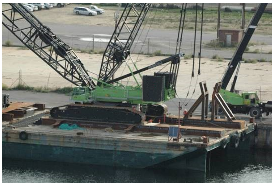
Photo showing an example of load spreading
