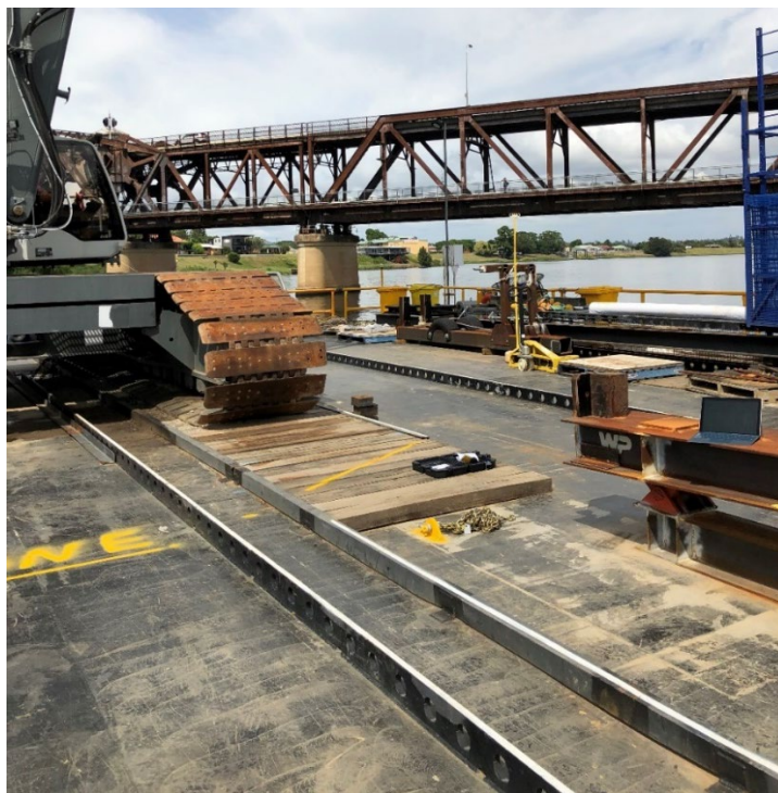
Figure 5b – Timber pads or matting needs to be secured on vessel deck
